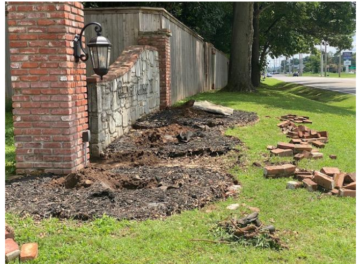
Volunteer Demolition & Cleanup
